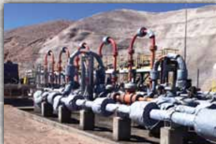
COOPER® Accuseal 8 inch, 1500 ASME Class Slurry Transport Valve in choke station pipeline for copper concentrate in Chile
