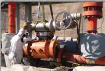
Valve removal for inspection
